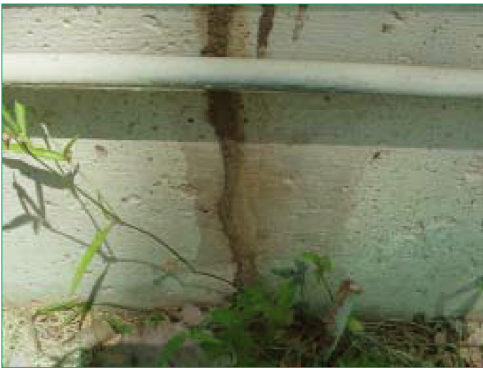
Figure 11. Shelter tube of an active termite colony.
